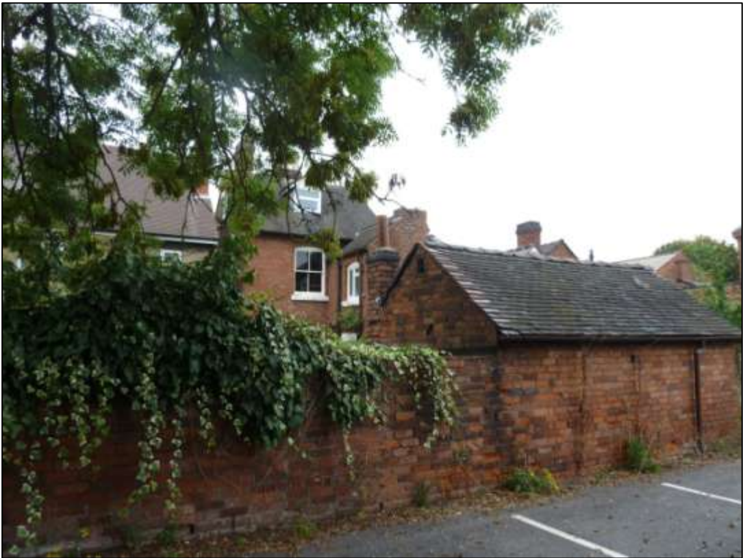
Figure 6 Remaining yard building to the rear of County Road
