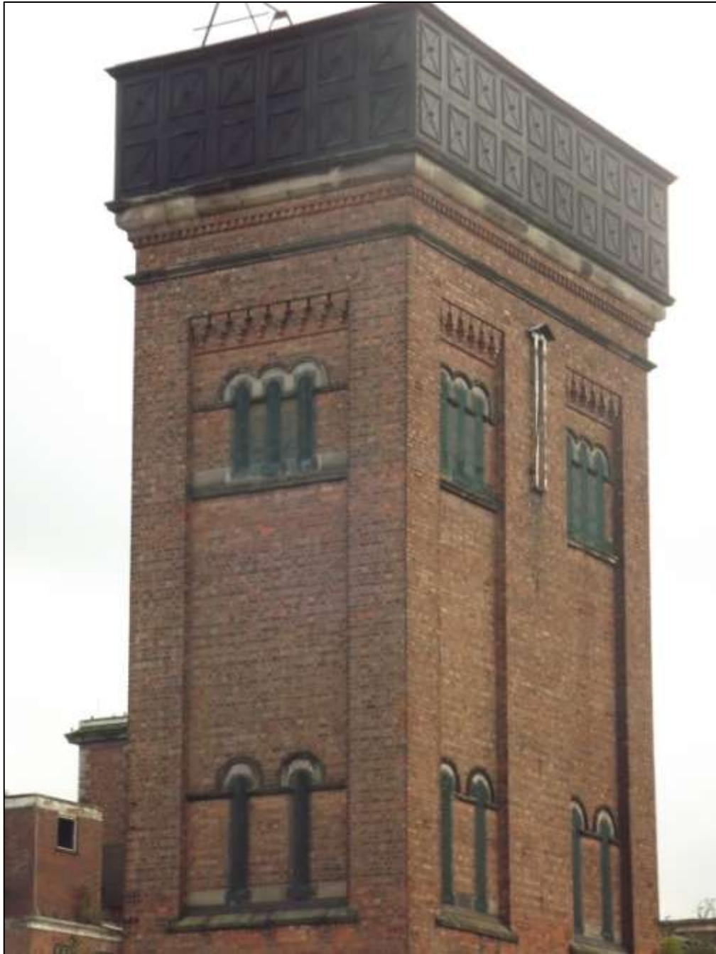
Figure 39 The Water tower
