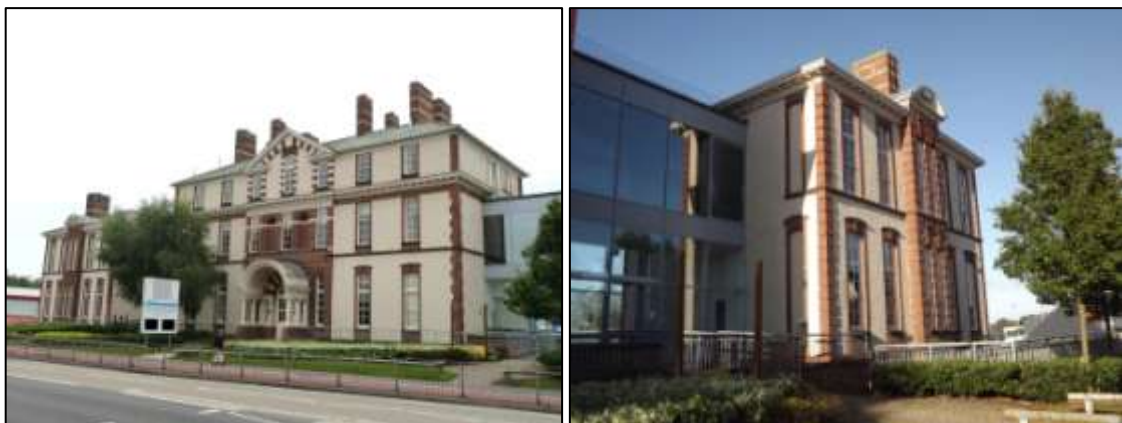
Figure 17 Staffordshire General Infirmary, east façade, and main entrance,
