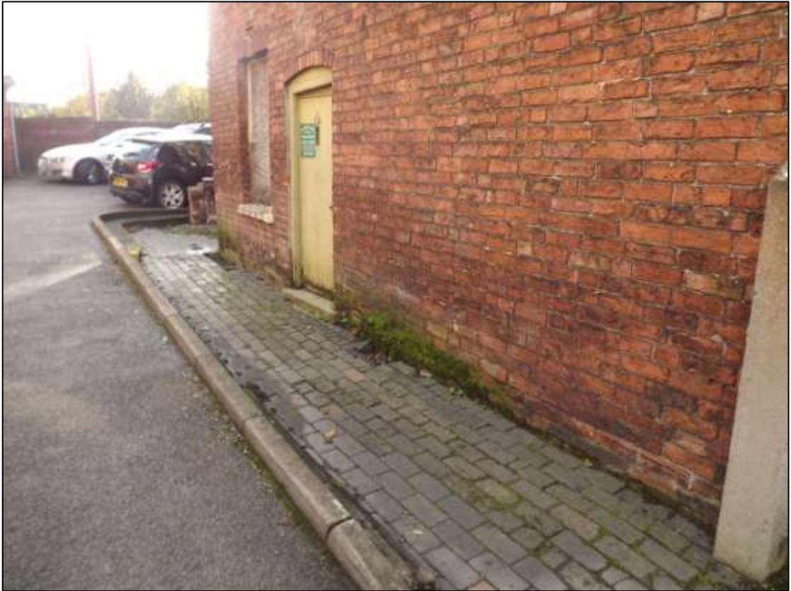
Figure 23 Blue brick remains to the side and rear of 14a County Road
