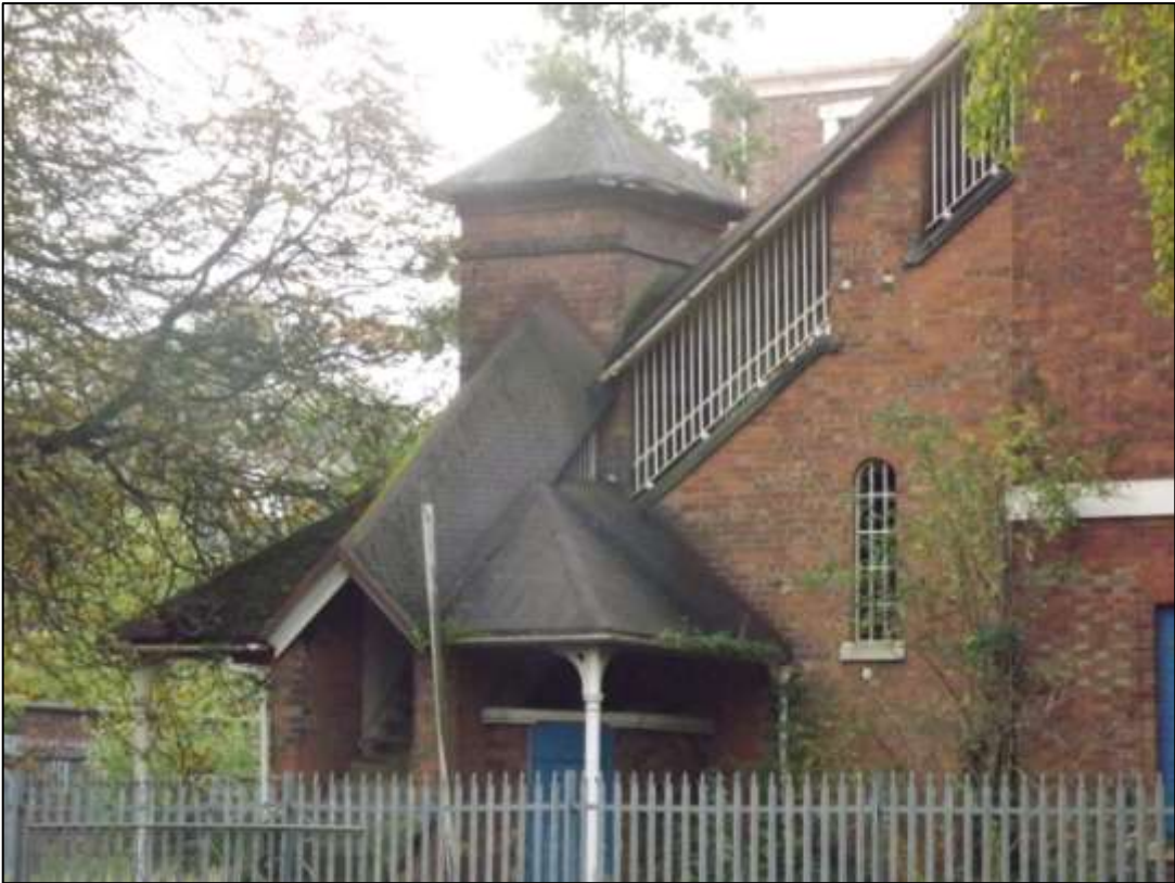
Figure 33 Covered walkway to “airing grounds” at the southeast of the south facade
