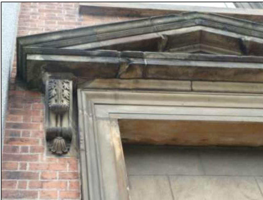
Figure 16 Stone detailing on the architrave to the entrance door
