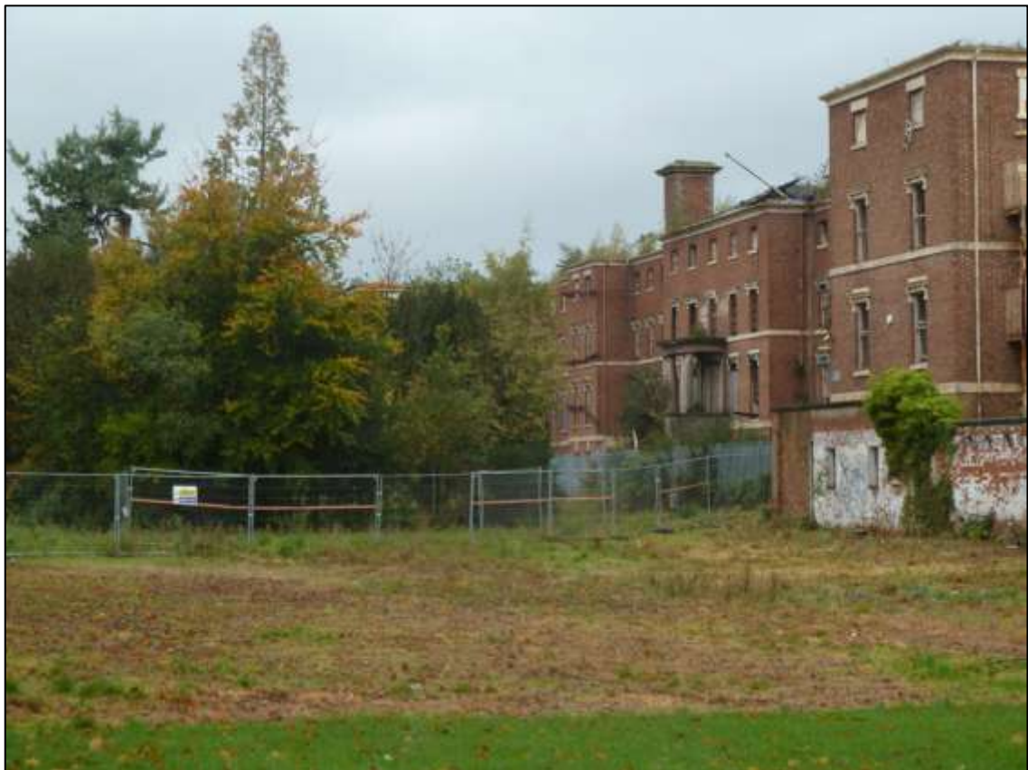
Figure 27 South facade, St George's Hospital
