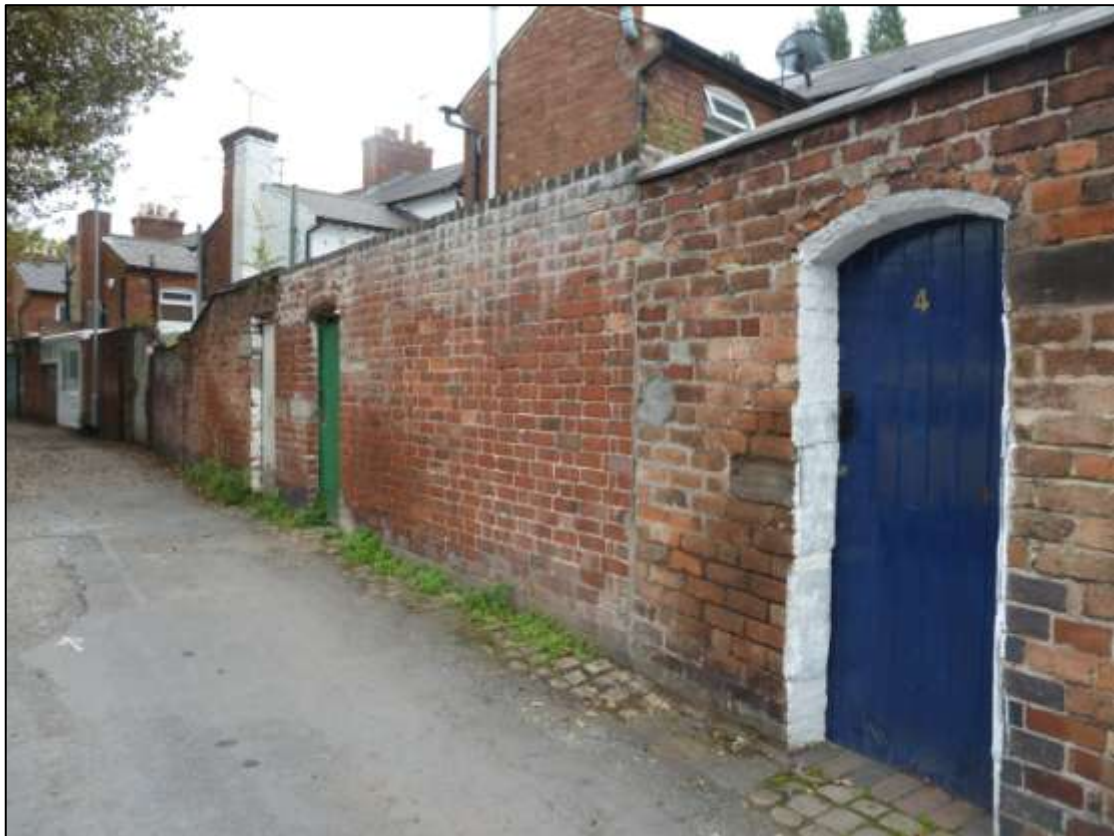
Figure 21 Setts along Chapel Terrace beneath modern paving surfaces
