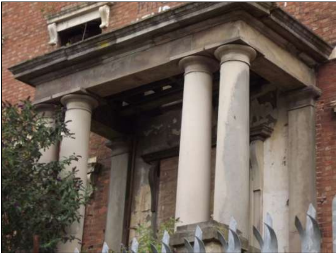
Figure 32 Tuscan portico to first floor, south facade, St George's Hospital
