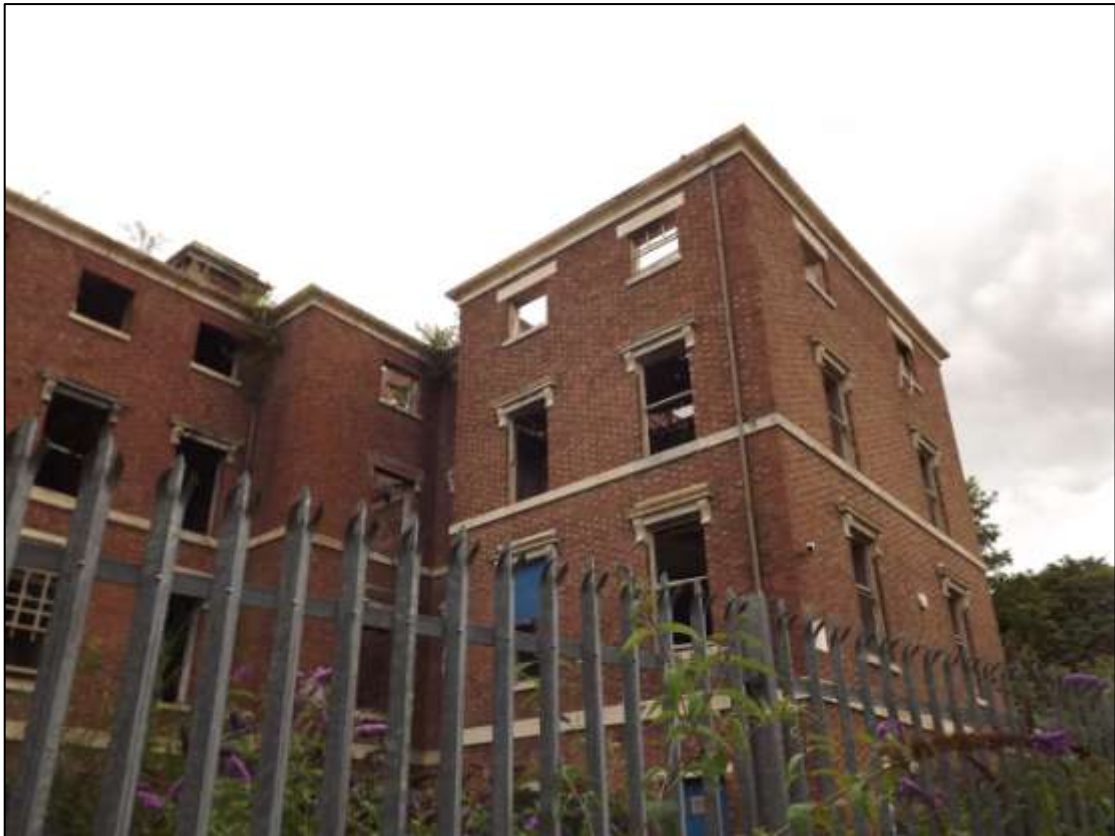
Figure 28 St George's Hospital south façade
