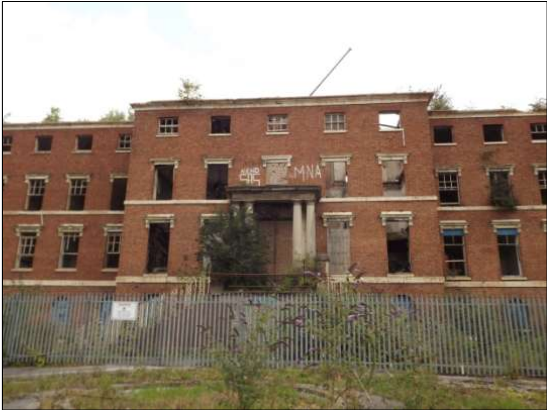
Figure 31 South facade, St George's Hospital
