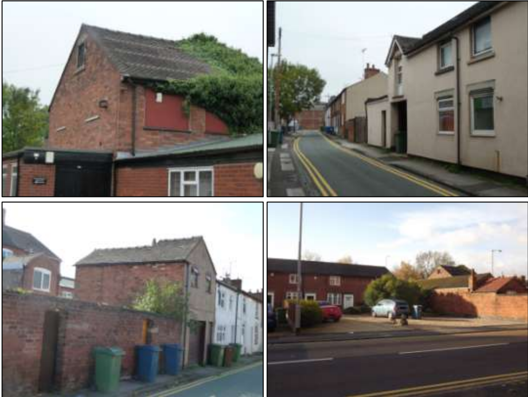
Figure 8 Top left: Former timber yard building, now part of Stonemason's yard. Right: The rectilinear former bakery on Foregate Street stretches onto Sash Street. The cart entrance remains on the ground floor, and former hayloft access remains on the first floor. Bottom left: Former workshop on Sash Street converted into a house. Right: 19th century terraces along Gaol Road and former timber yard buildings to right
