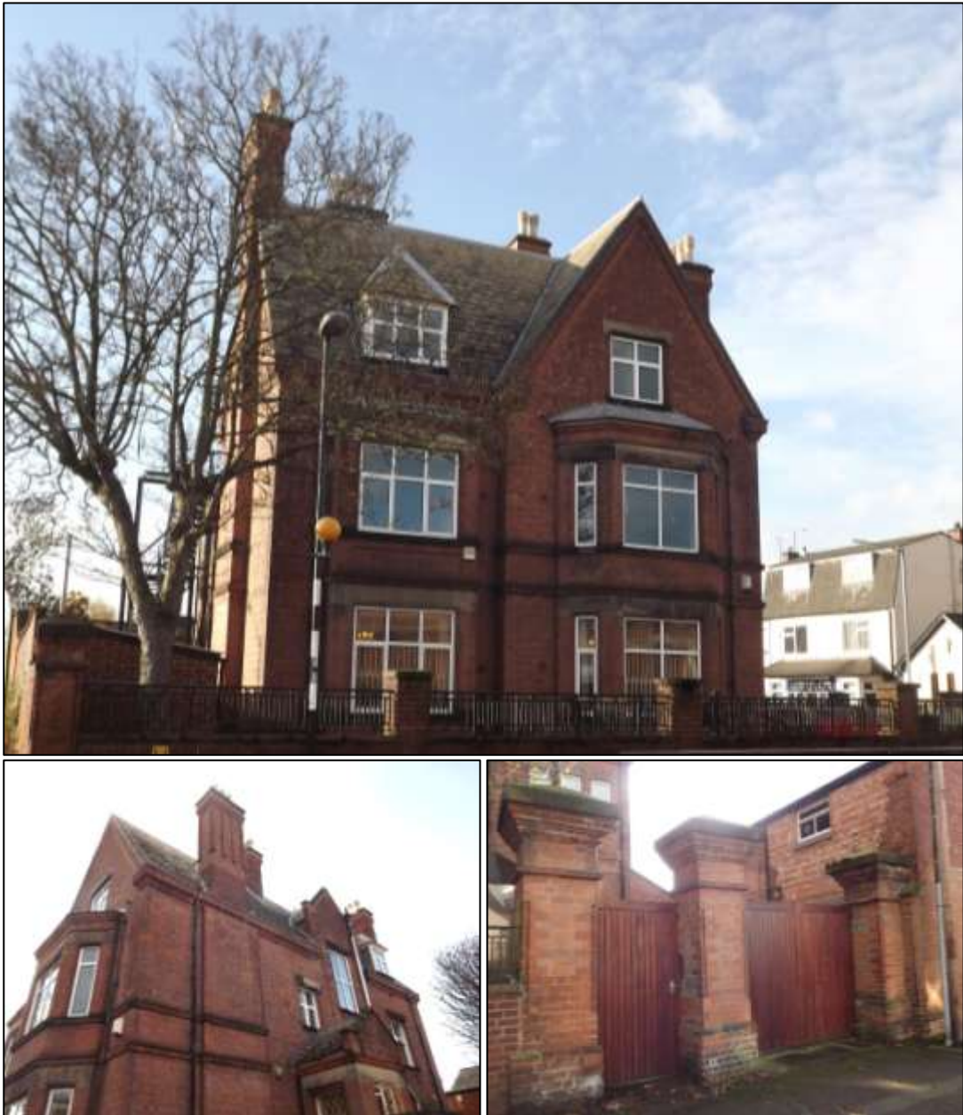
Figure 11 21 Goal Road with Neo Tudor and Domestic Revival elements. The large gate piers with moulded brickwork give the building presence in the street scene
