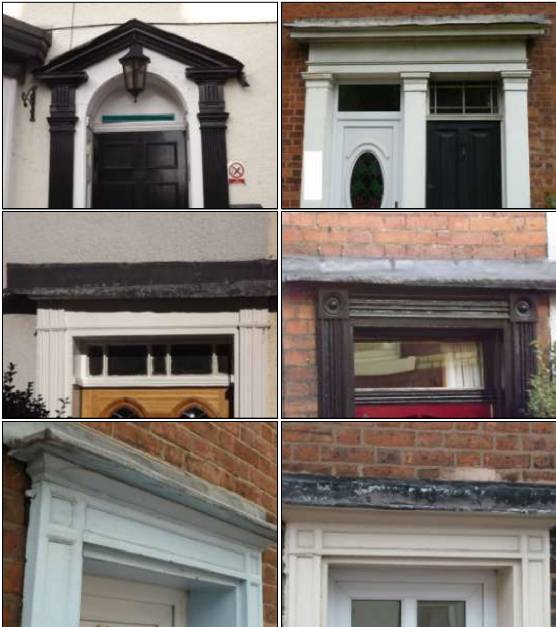
Figure 14 Fanlights and door cases on Chapel Terrace and County Road
